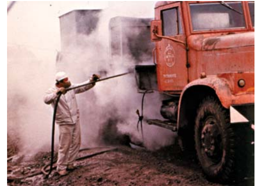
Decontamination of machinery during the liquidation of the accident
