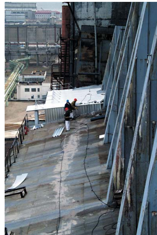
Sealing the Shelter roof
