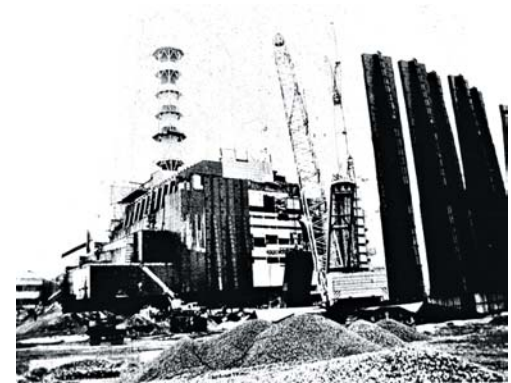
Erection of the western buttress wall
