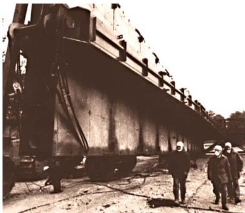
The Shelter's Mammoth beam shortly before being lifted into position over the destroyed unit
