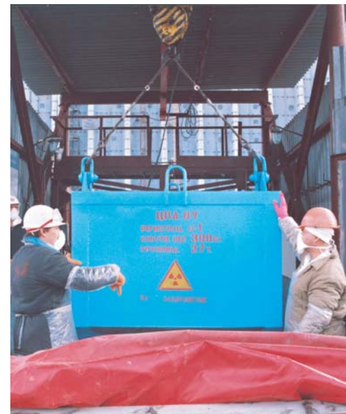
Container of Shelter-derived radioactive waste prior to disposal
