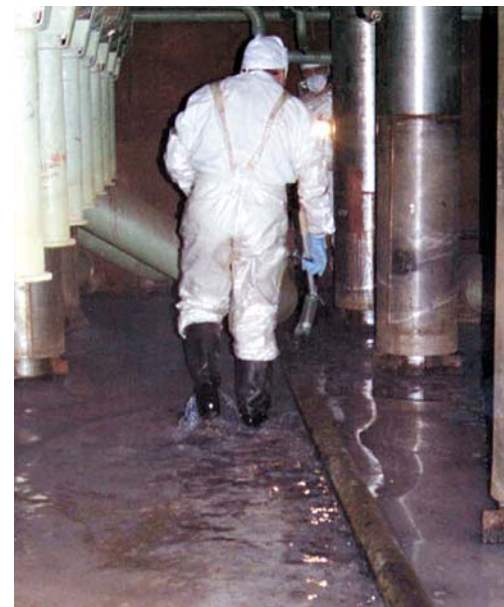
Water ingress presents a hazard for structures and radioactive materials of the Shelter Object
