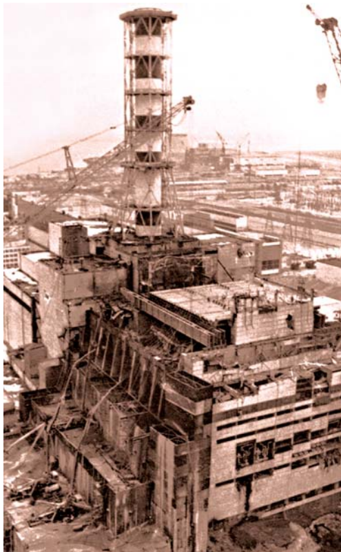
Construction of the Shelter Object northern cascade wall
