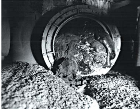
Radioactive hazard of the Shelter. Frozen fuel lava
