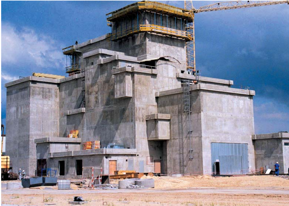
Construction of a new spent fuel dry storage facility at the ChNPP
