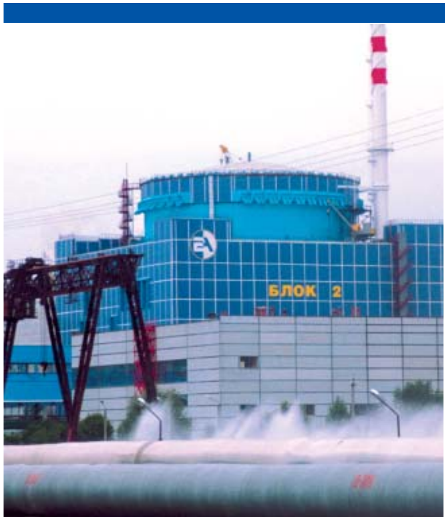
▲ New Unit of Khmelnytsk NPP. The Ukrainian Government plans to support construction of nuclear units
