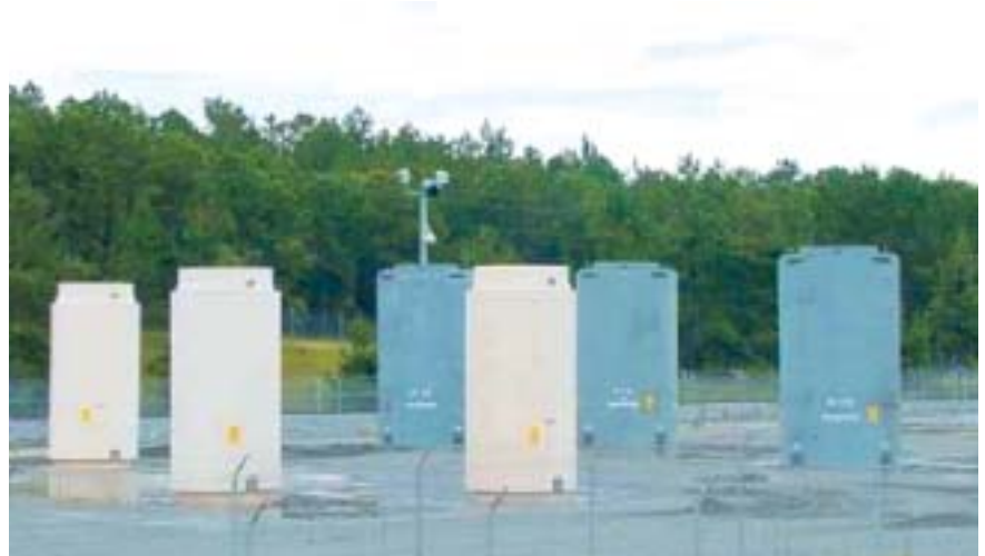
▼ Spent nuclear fuel dry storage in containers
